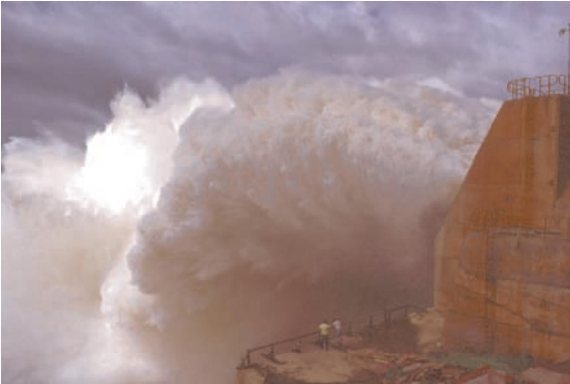
One of the world's largest dams — the Itaipu hydroelectric plant in Brazil. The future of such projects is called in question by a new report
